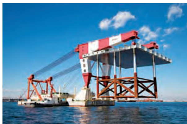
Piled-elevated platform during construction. The runway was created after connecting the component to a steel jacket.
