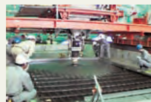
Test pouring of the concrete slab
