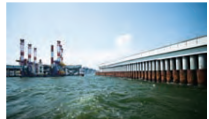
Wave-absorbing seawall during construction. 229 concrete pillars were installed for the seawall (428 m) on the reclaimed island side.
