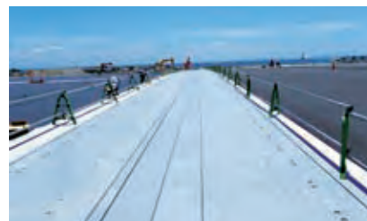
“Roller-shutter type” expansion joint (linking the reclaimed island and piled-elevated platform of the runway) during construction
