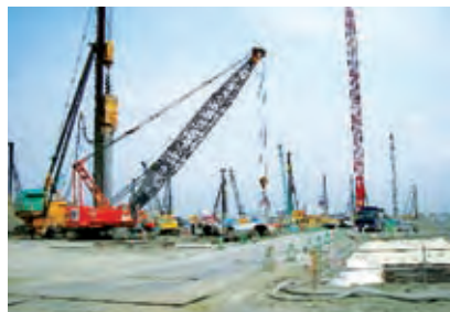
Steel pile construction work
