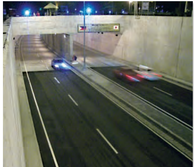
Cebu South Coastal Road, Philippines
