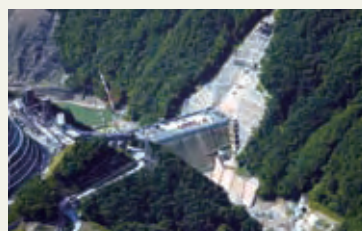
View of the entire worksite
