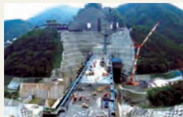
Casting the concrete body of the dam
