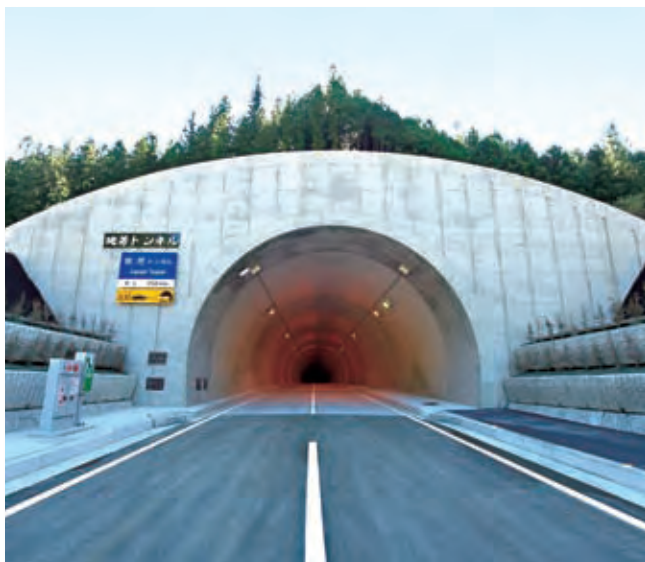
Jiyoshi Tunnel, National Highway No. 440
