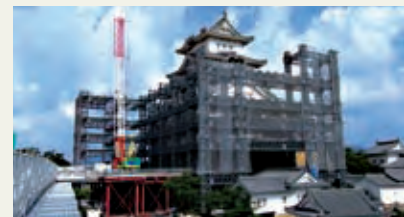
Himeji Castle under restoration
