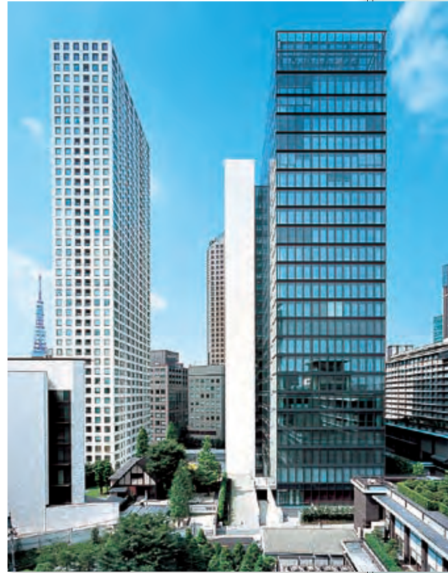
Toranomon Towers Office (Under operation since 2006)
