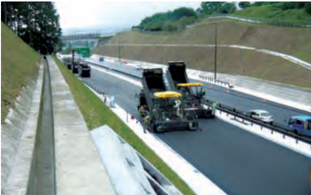
Road paving work on the Izu Jukan Tokura Road (Constructed by Kajima Road Co., Ltd.)
