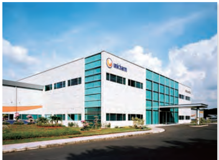
Unicharm No. 2 Indonesia Plant
