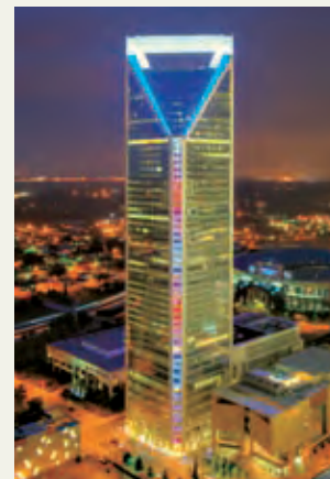
Duke Energy Center (Constructed by Batson-Cook Construction)
