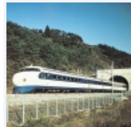
1963 New Tanna Tunnel
