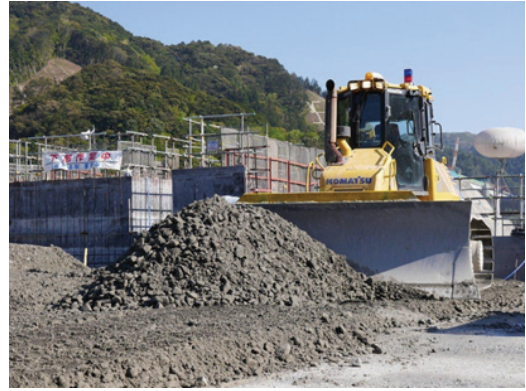
Photo 4 RCD ダム工事での自動運転状況 (Situation of Automatic Operation in Dam Construction)
