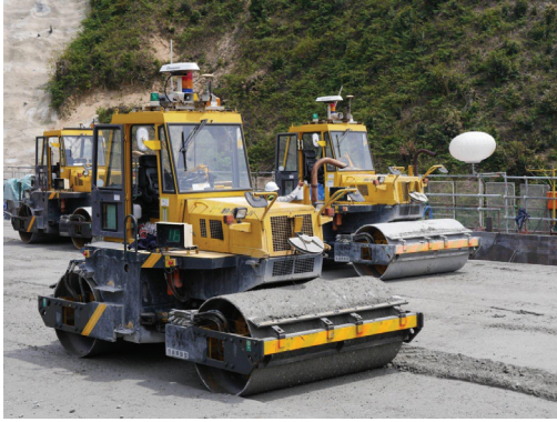
Photo 2 同時施工の状況 (Situation of Simultaneous Construction)
