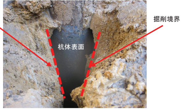
Photo 4 掘削結果 (Excavation Results)
