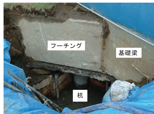
Photo 1 杭頭調査事例 (Example of Pile Investigation)
