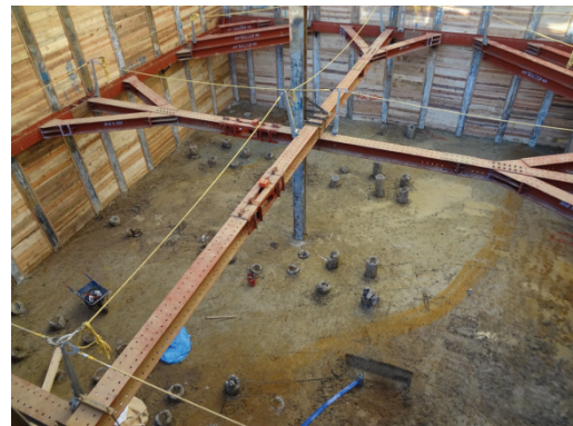
Photo 2 実験場所 (General View of Test Site)
