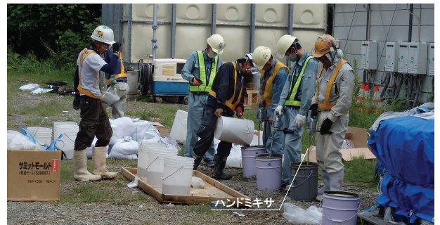
Photo 2 凝結遅延モルタルの練混ぜ状況 (Status of Mixing Mortar)
