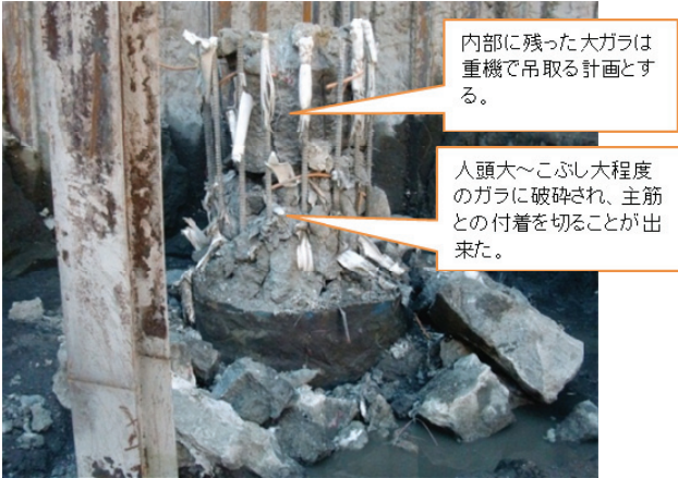
Photo 10-1 破砕後の状況 (Demolition Result)
