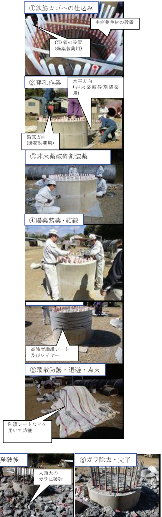
Fig.2 作業手順 (Work Procedure)
