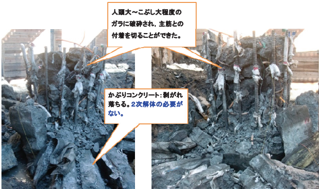
Photo 10-2 破砕後の状況 (Demolition Result)
