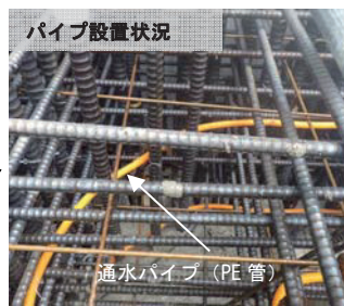
Photo 3 PE 管設置状況 (Pipe Location)
