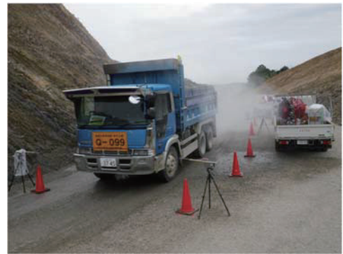
Photo5 ダンプ走行時の噴霧状況 (Spray Situation at the Time of the Dump Traveling)
