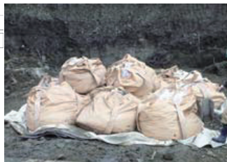
Photo 6 防護完了 (Appearance of Protection)
