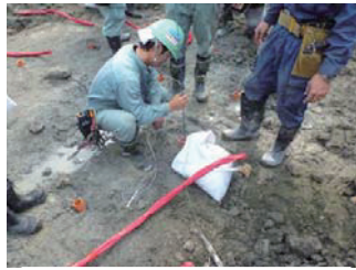
Photo 5 装薬・結線 (Setting Explosives)
