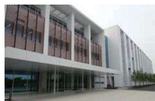
Fig. 8 建物外観 (Outline of Building)
