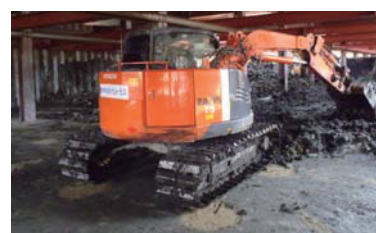
Photo 1 施工状況 (Excavation after SCP Ground Improvement)
