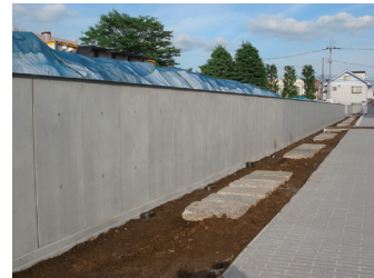
Photo 5 外構擁壁 (再生細骨材M) (Appearance of Outward Wall)
