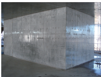
Photo 3 柱・壁 (再生細骨材H) (Appearance of Pillar and Wall)
