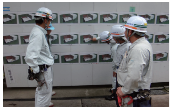
Photo 1 朝礼看板への施工ステップの掲示 (Example of Construction BIM in Construction Site)
