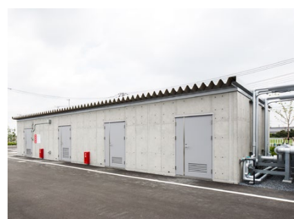
Photo 7 付属舎棟施工後の外観 (Exterior of Machinery Building)
