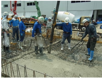
Photo 3 基礎耐圧盤打設状況 (Placing of Foundation and Pressure Slab)
