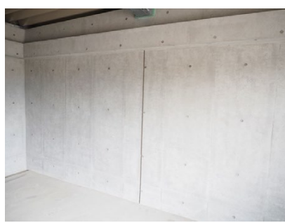
Photo 6 壁部施工後の状況 (Appearance of Wall)
