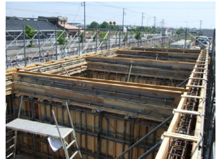
Photo 4 壁部施工状況① (Placing of Wall ①)
