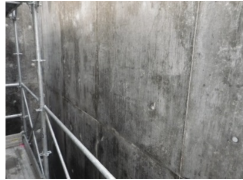
Photo 5 脱型後の外観 (Concrete Surface After Demolding)
