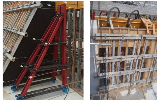
Fig.13 埋設鋼材の設置状況 (Installation of Embedded Steel Materials)
