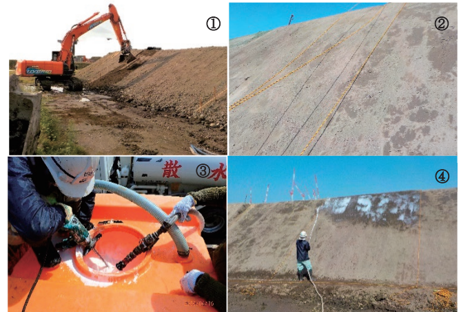
Photo 4 施工試験準備 (Preparation of Construction Test)
