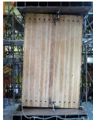
Photo 2 損傷状況 (Damage Appearance of S-M12)
