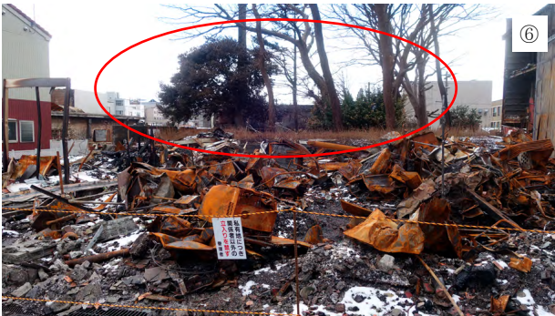
Photo 4 延焼阻止に寄与した樹木 (Trees that Helped Stop the Spread Fire)
