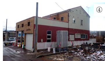
Photo 2 延焼を免れた住宅 (Houses that Escaped the Fire Spread)
