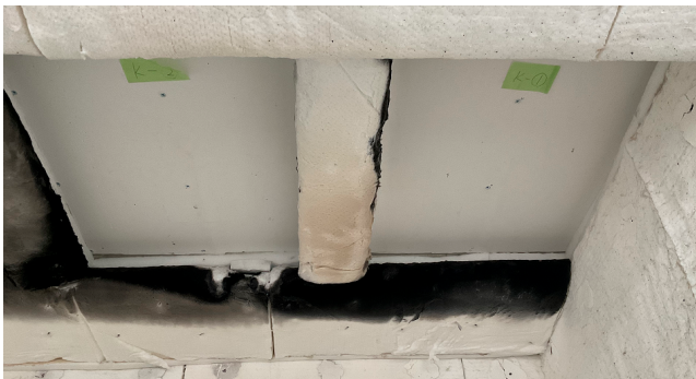
Photo 6 試験体設置状況 (Test Situation of Heating Test)
