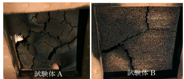
Photo 5 試験後の状況 (Specimen after Heating Test)
