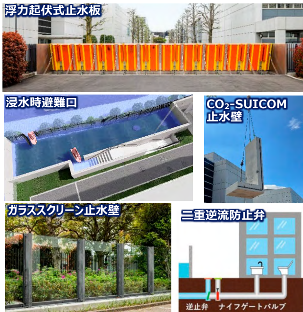
Fig.8 特徴的な水防設備 (Distinctive Flood Prevention Facilities)
