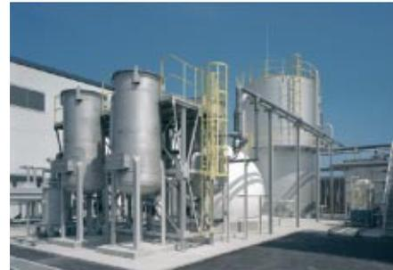
The facility was constructed as a part of the Field Evaluation Project in the Ministry of Environment's "Global Warming Prevention Measures Program" under its auspices. The newly constructed facility microbiologically converts organic waste to methane-rich biogas that is then reformed to hydrogen and supplied to the PAFC for power generation.
